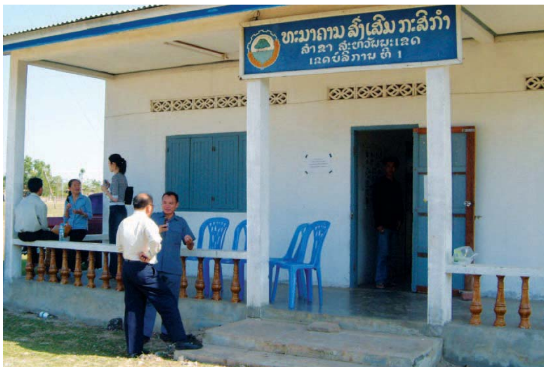
APB's subservice unit in Savannaket Province
